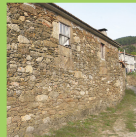
House of the priest and teacher Manuel da Lixa, a Latinist of repute. The photographic record shows the house prior to restoration.
